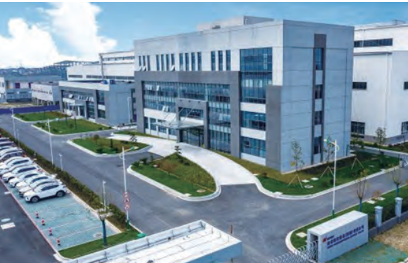
Neway Precision Forging(Liyang),.LTD Main products: Hammer forging, annular forging Office area: 3,000 sqm Work shop: 30,000 sqm
